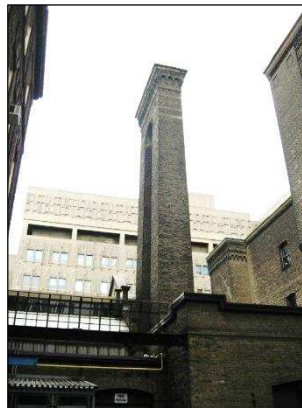
Figure 2.11: Exhaust chimney outside the Mechanical Engineering building, University of Toronto.
